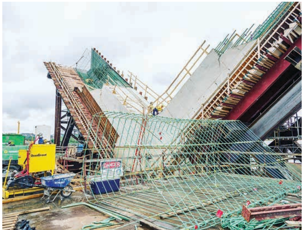
Partially completed V-piers with rebar
